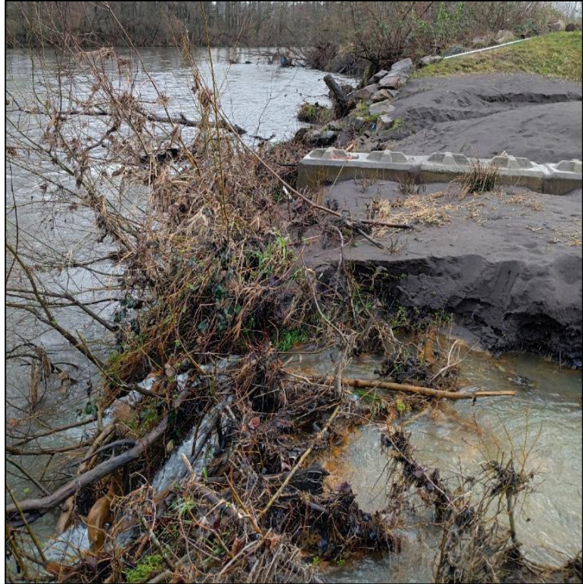
Figure 4-11. Concentrated flow spilling over, eroding, and undercutting vegetated bank. Photo taken on March 15, 2022, NHC.
