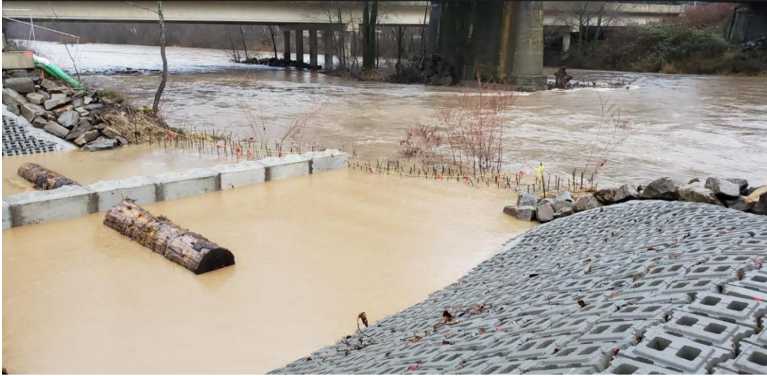
Figure 4-19. Photo above from December 2019, showing flooding as well as willow wands and large boulders on the top of riverbank at the outside edge of the outfall structure. Photo below is from December 2022, showing the riverbank erosion, willow wands stripped away, boulders falling down the slope into the river, and deep sand deposits.
