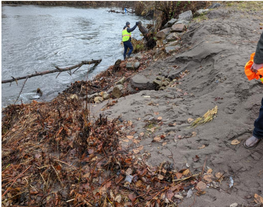
Figure 4-19. Photo above from December 2019, showing flooding as well as willow wands and large boulders on the top of riverbank at the outside edge of the outfall structure. Photo below is from December 2022, showing the riverbank erosion, willow wands stripped away, boulders falling down the slope into the river, and deep sand deposits.
